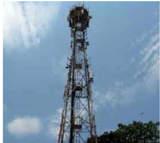
Fig. 1.2.2(ii): A telecom tower
